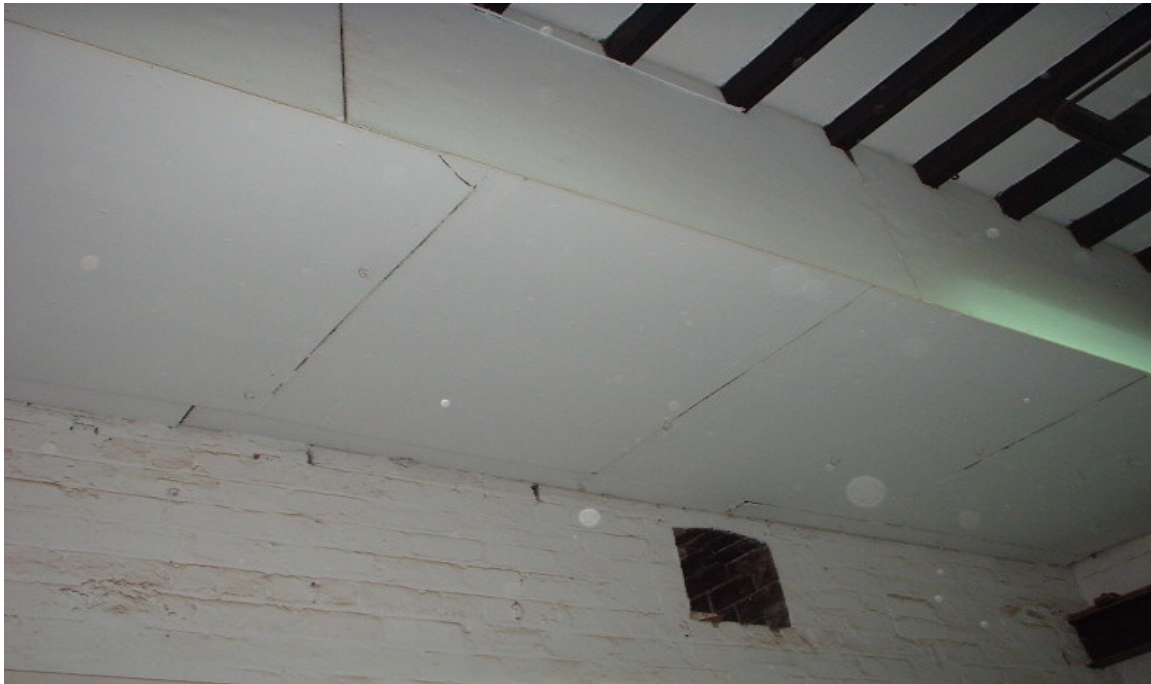
Asbestos Cement Boards @ Sub-basement, Woodwork Workshop, Bulkhead
