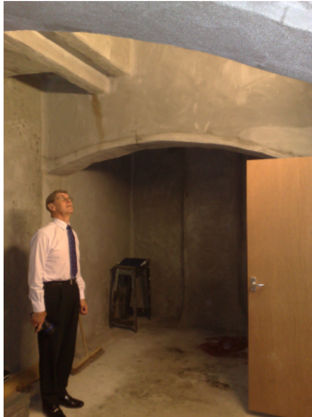
Fig. 12 – Potential plant space location – Ex-Timber Store at Basement Level
