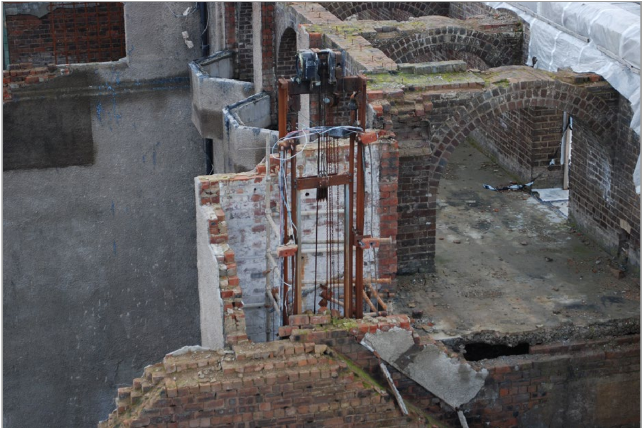
Figure 21 – Top of lift mechanism, west side
