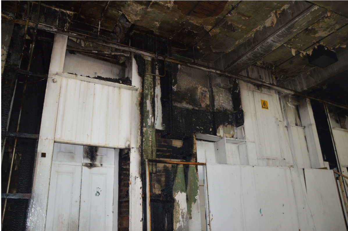
Photo 12. Studio 31 Ground floor. To right of door fire spread up vertical void
