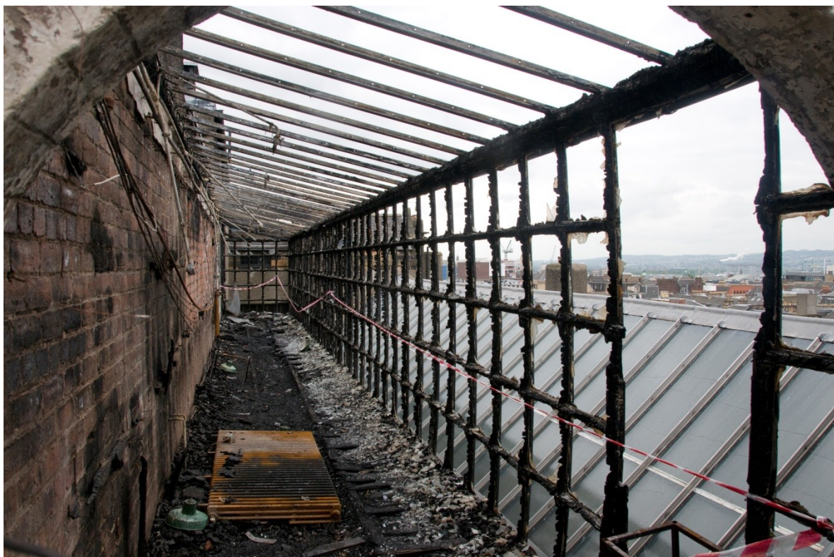
Photo 20. 2 nd floor Hen run south elevation, looking east.
