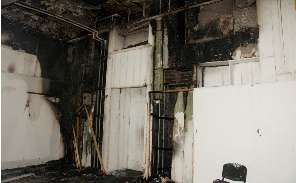
Photo 10. Studio 31 Ground floor. Fire spread vertically via voids either side of door. Note V pattern. Less damage in this area as fire spread to floor above at wall/ceiling junction.
