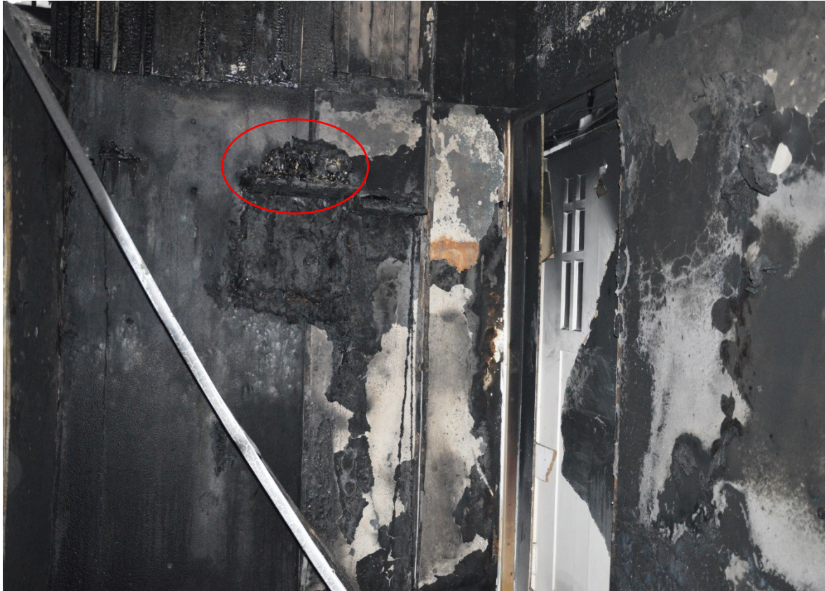
Photo 4. Within studio 19, the student display area, south wall, projector circled
