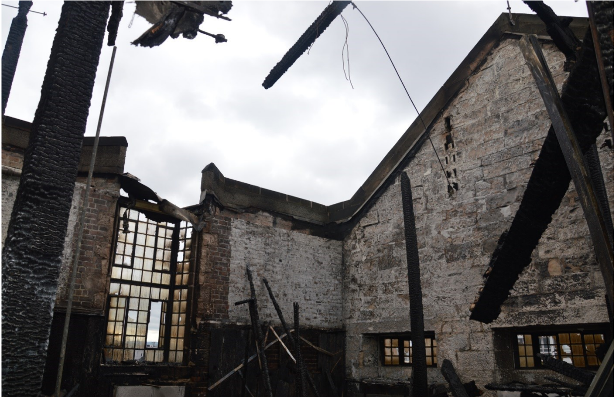
Photo 16. 2 nd floor Studio 58 looking south
