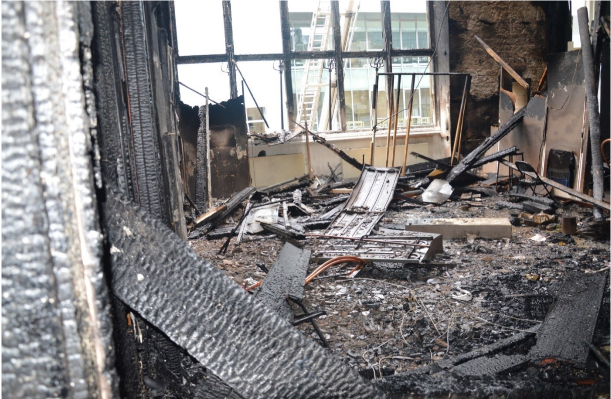
Photo 18. First floor studio 45, looking north onto Renfrew Street
