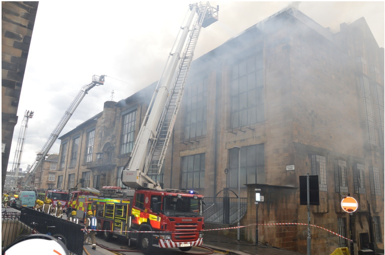
Photo 24. Aerial Rescue Pumps at work on north side of building
