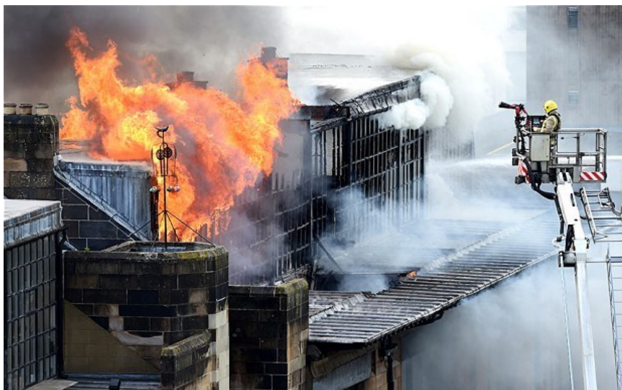
Photo 21. Professor Studios on 2 nd floor north elevation totally involved in fire. Image courtesy of Craig Watson SNS Group.
