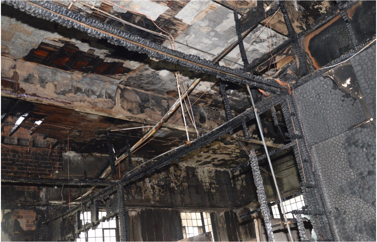
Photo 14. Ground Floor Studio 32 looking south west.
