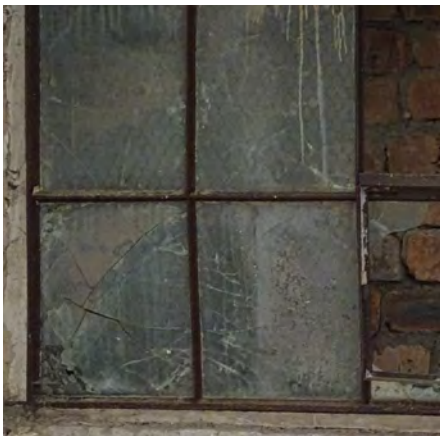
Steel framed window and glazing
