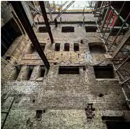
West external wall of offices, toilets and museum
