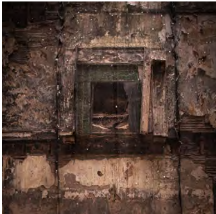
Caretaker's House fireplace
