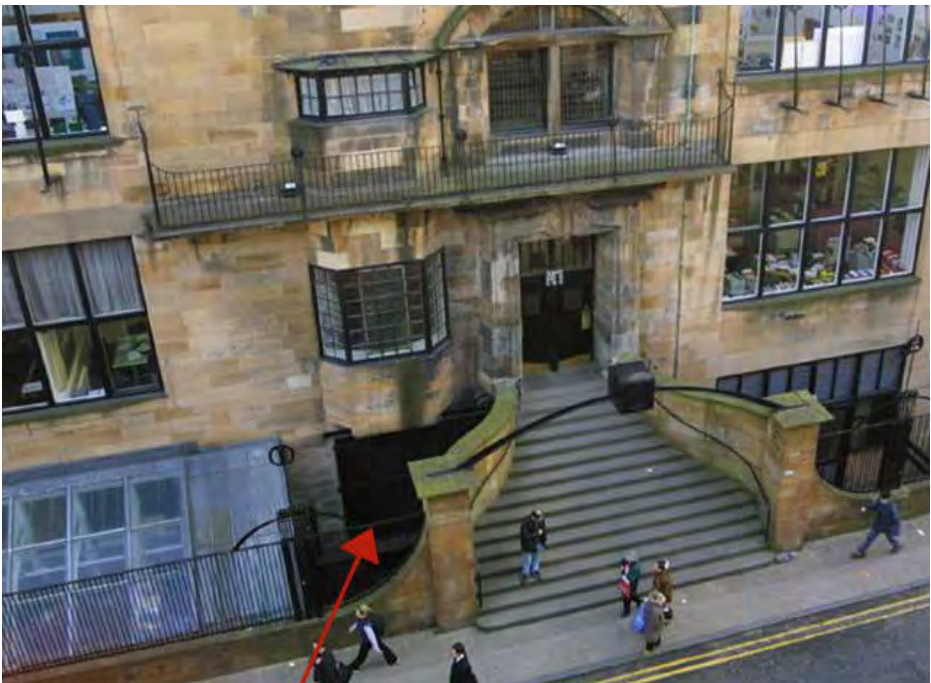
Potential location for intervention to allow level access, adjacent to the main entrance on Renfrew Street
