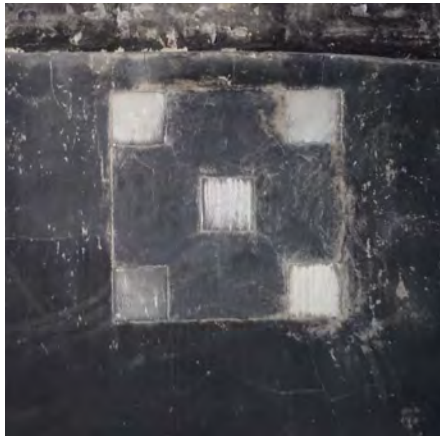
Tiles in the East Stairwell
