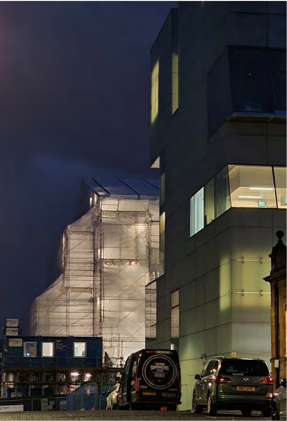
Shoring scaffold, viewed from Dalhousie Street
