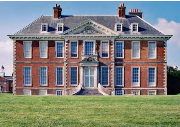
Uppark House, reinstated
