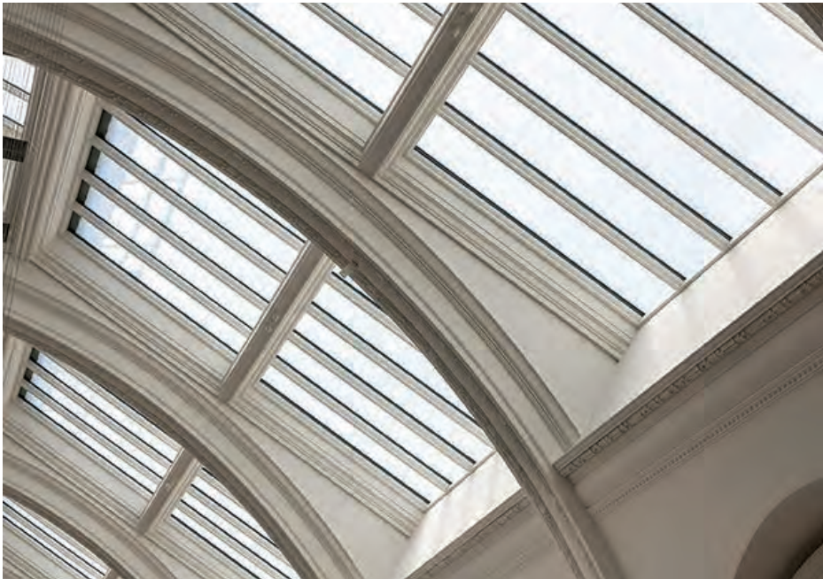
Double glazed patent glazing at the V&A Kensington
