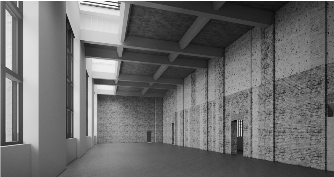
First Floor studio with internal wall insulation
