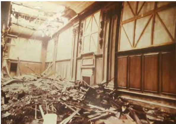
Hampton Court Palace, fire damaged
