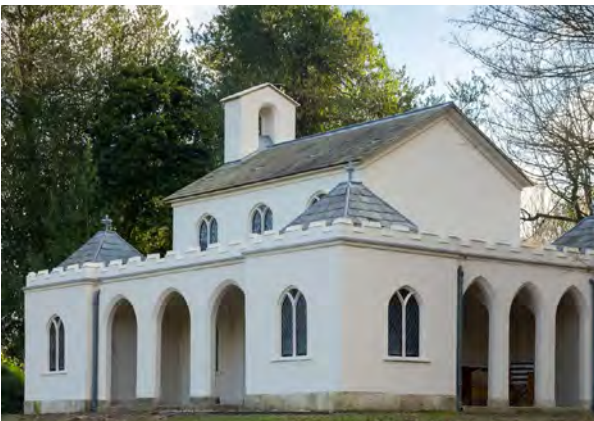
Cobham Dairy, reinstated
