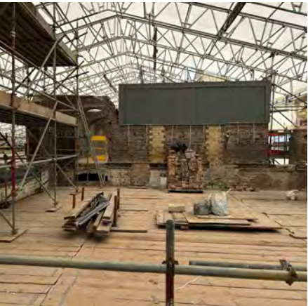
Internal wall between studio 58 and stair
