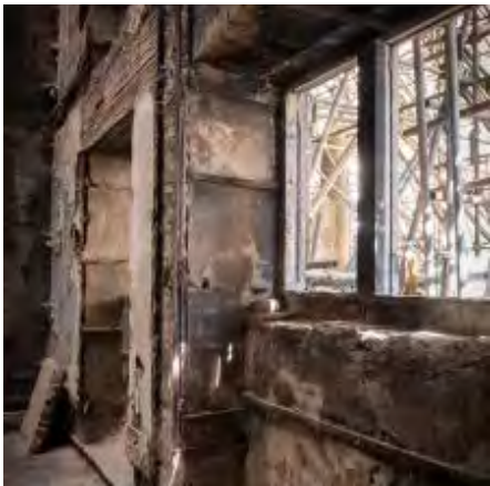
Windows at Caretaker's House
