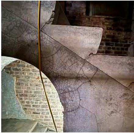
East Stairwell - concrete treads and plaster
