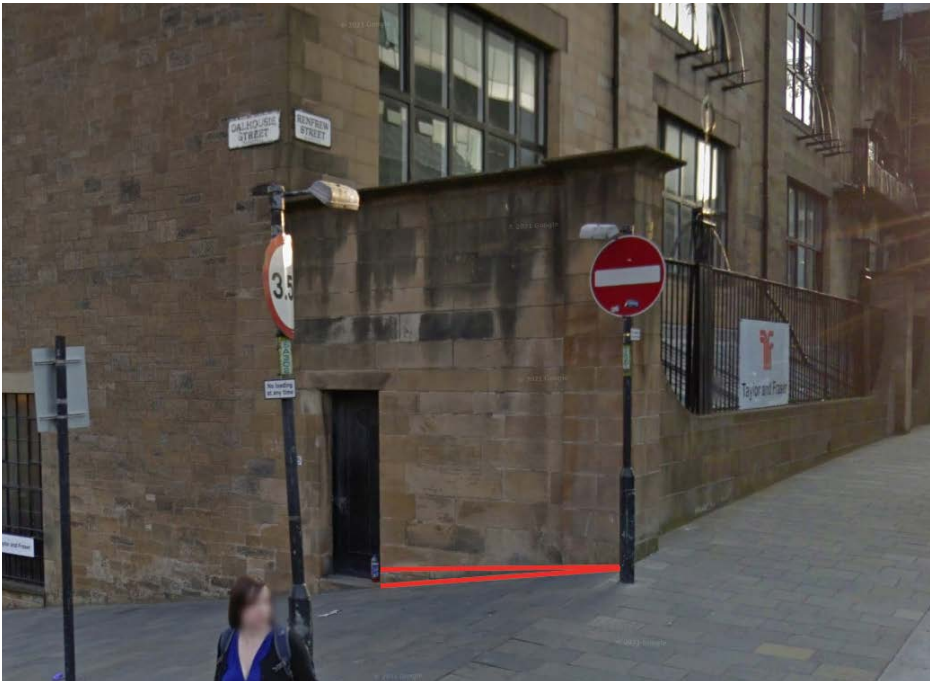
Potential location for intervention to allow level access, on Dalhousie Street
