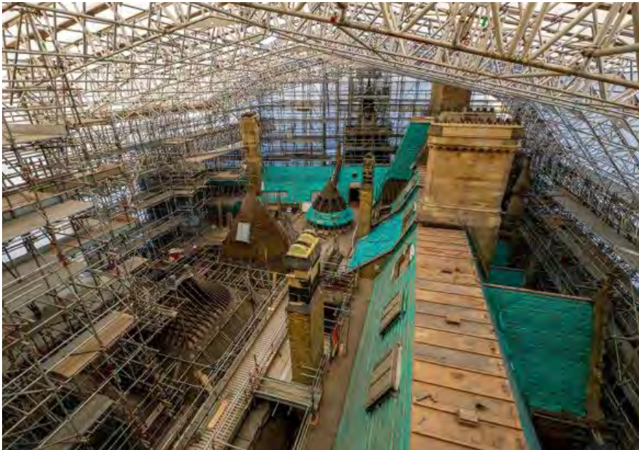
Manchester Town Hall, restoration
