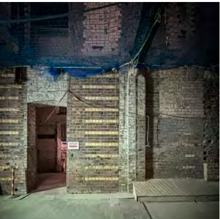
Core wall at basement
