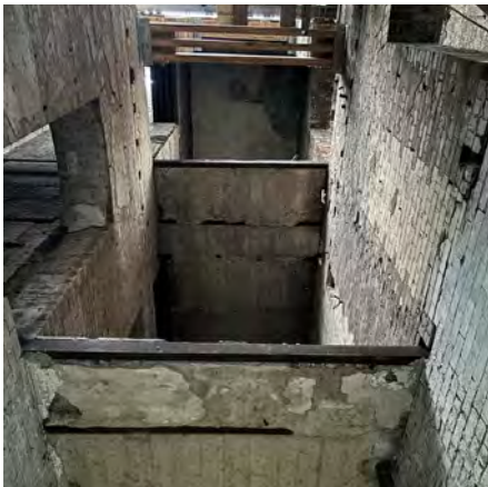
Concrete corridor floors
