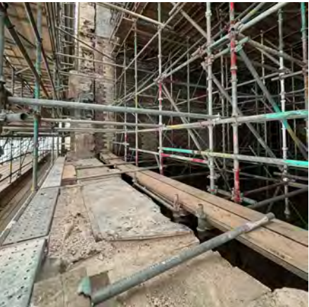
Window cill level of library
