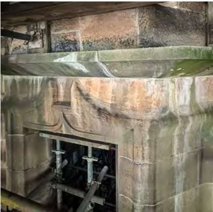
Stone at window head on East elevation
