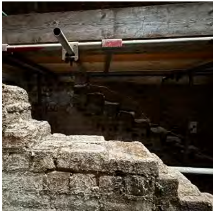
Seating for main stair from ground to basement
