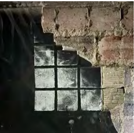
West stair tiling
