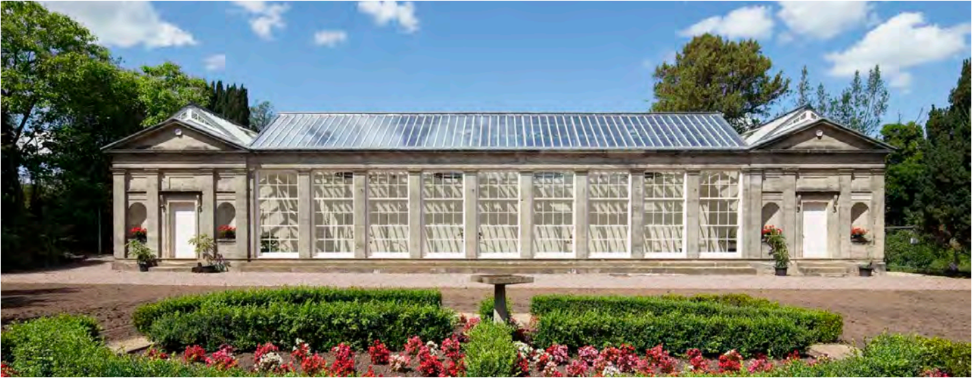
Ingestre Orangery after restoration
