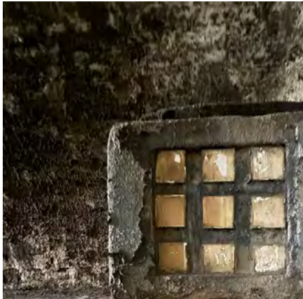
Tiles in the sub-basement
