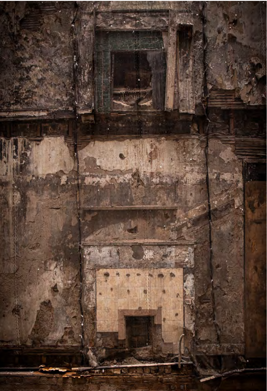
Fireplaces in the Caretaker's House
