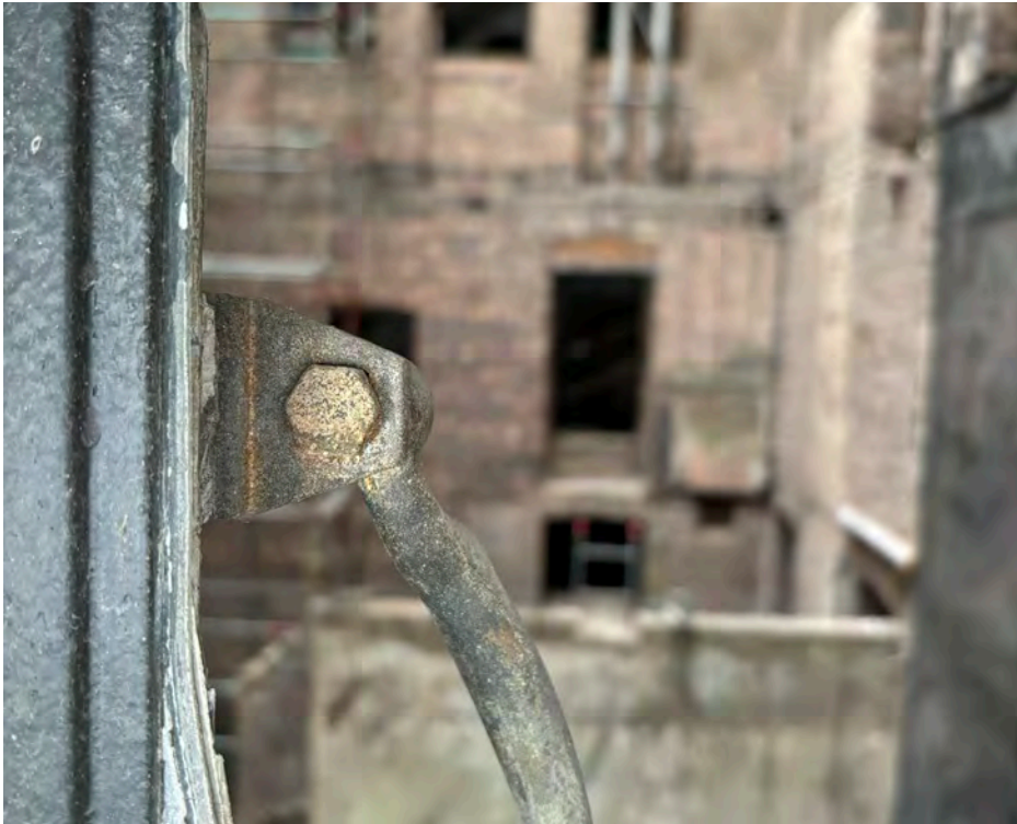
Type 1 - Caretaker's house - leaded, steel framed (handle remains)
