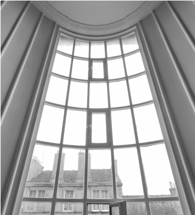
Type 4 - design room - curved timber frame
