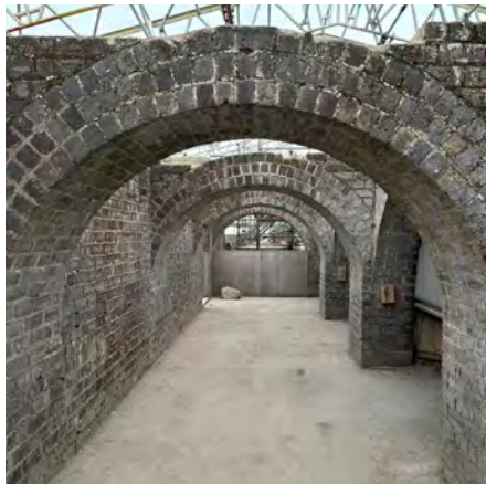
Brick arches at loggia
