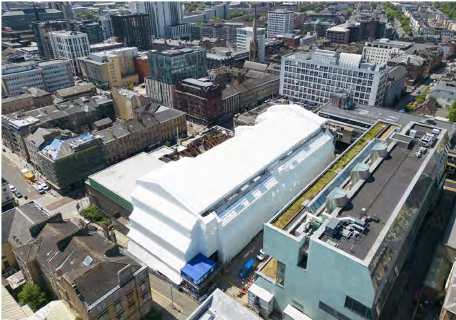
In 2024 the building was shrouded in scaffold. The wrap was removed from the walls in April 2025
