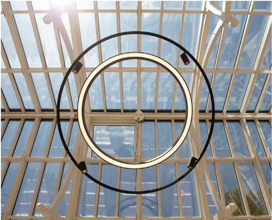
Ingestre Orangery after restoration
