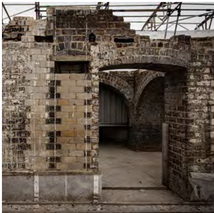
Brickwork at second floor
