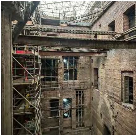
West and North Brick walls to Mackintosh Room
