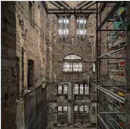
Wall at Mackintosh Room and Caretaker's House
