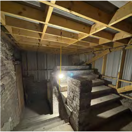
Top of East Stair
