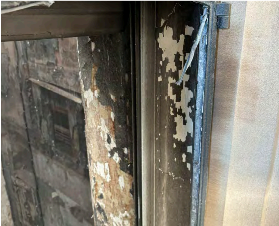
Type 1 - Caretaker's house - leaded, steel framed (image shows alter added frame of secondary glazing inside)
