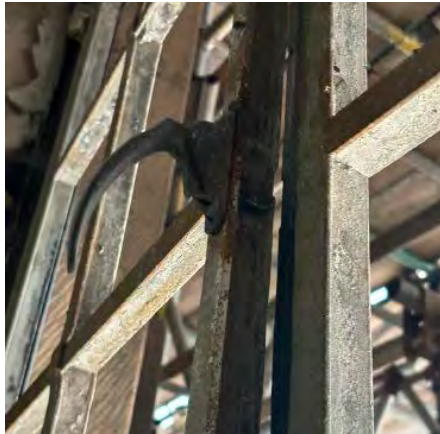
Window ironmongery on West Elevation
