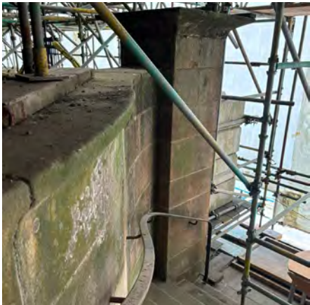
Entrance steps wall and handrail
