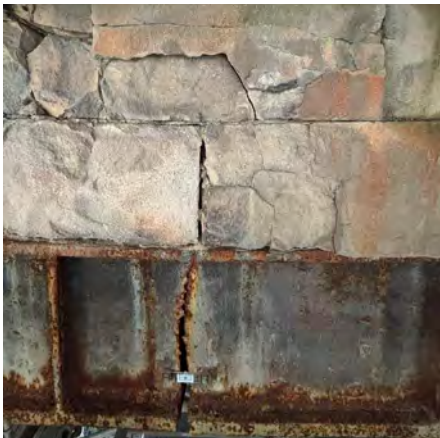
Cast iron window lintel at Ground Floor Studio
