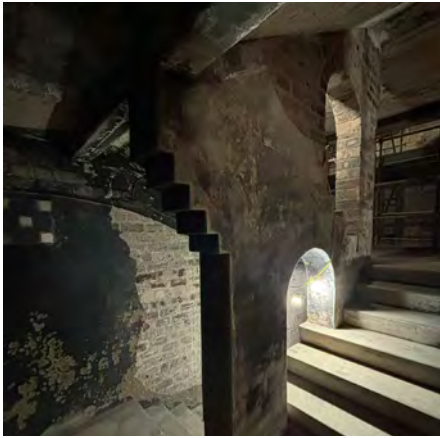
East Stairwell - surviving tiling and plaster
