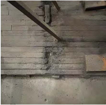
Surviving timber strip flooring at Basement
