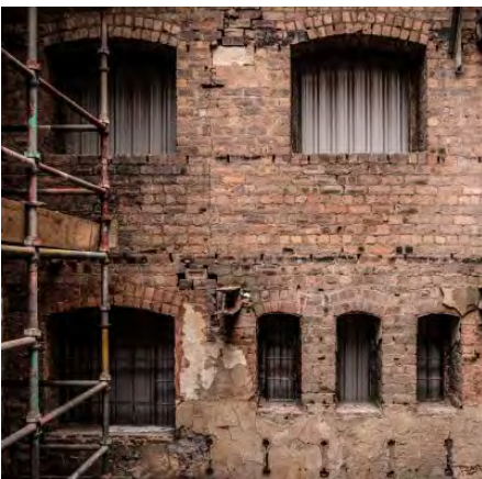
Window openings to toilets and offices
