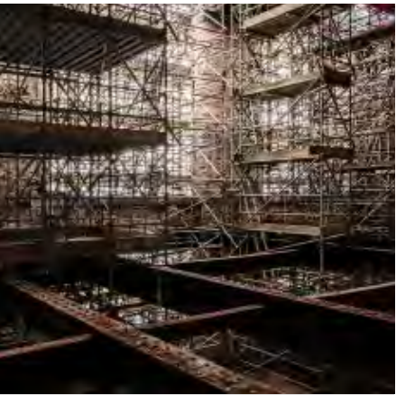
Cast steel beams and North elevation in studios
