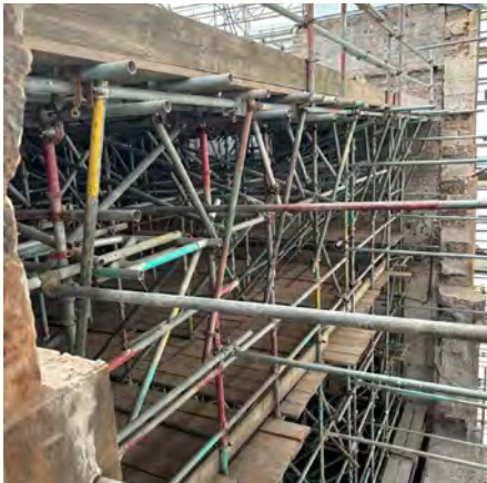
Removed west wall of library
