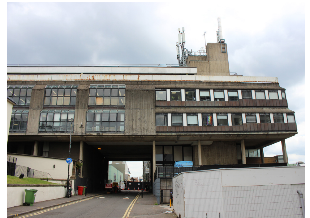
Brutalist Bourdon building crosses Renfrew Street and obscures views of the site
