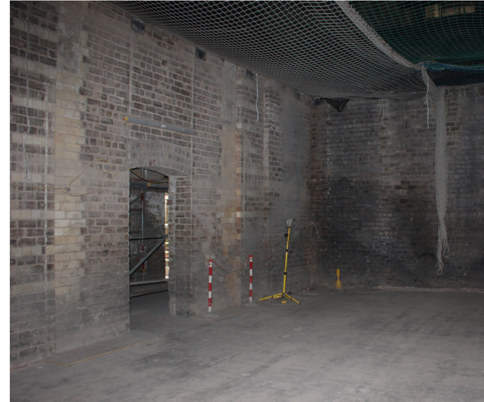
Brick partition walls in basement, yellow bricks indicate flues
