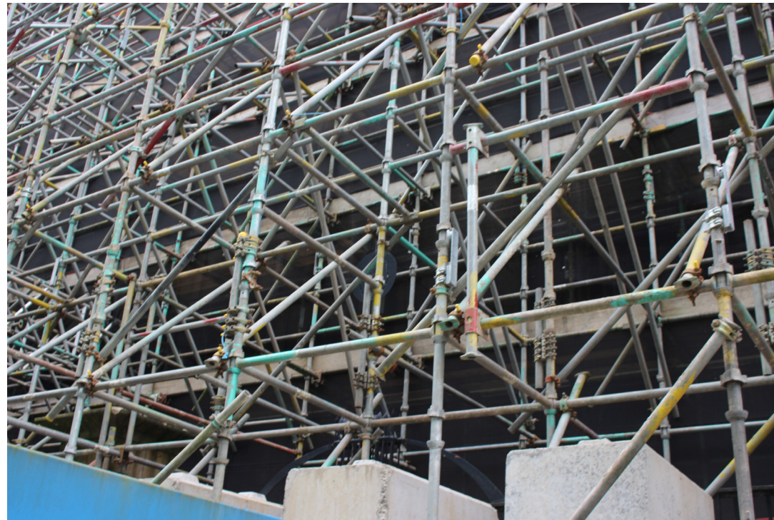
Original floral railings and motif of north front survived fire, visibility limited by scaffolding.
