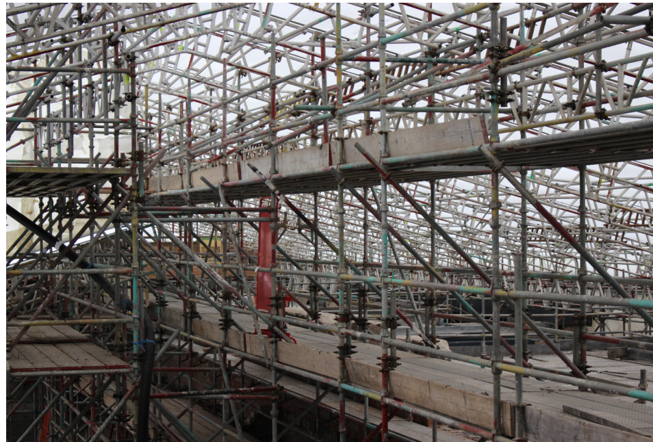
Mass of scaffolding obscures the form of the roof
