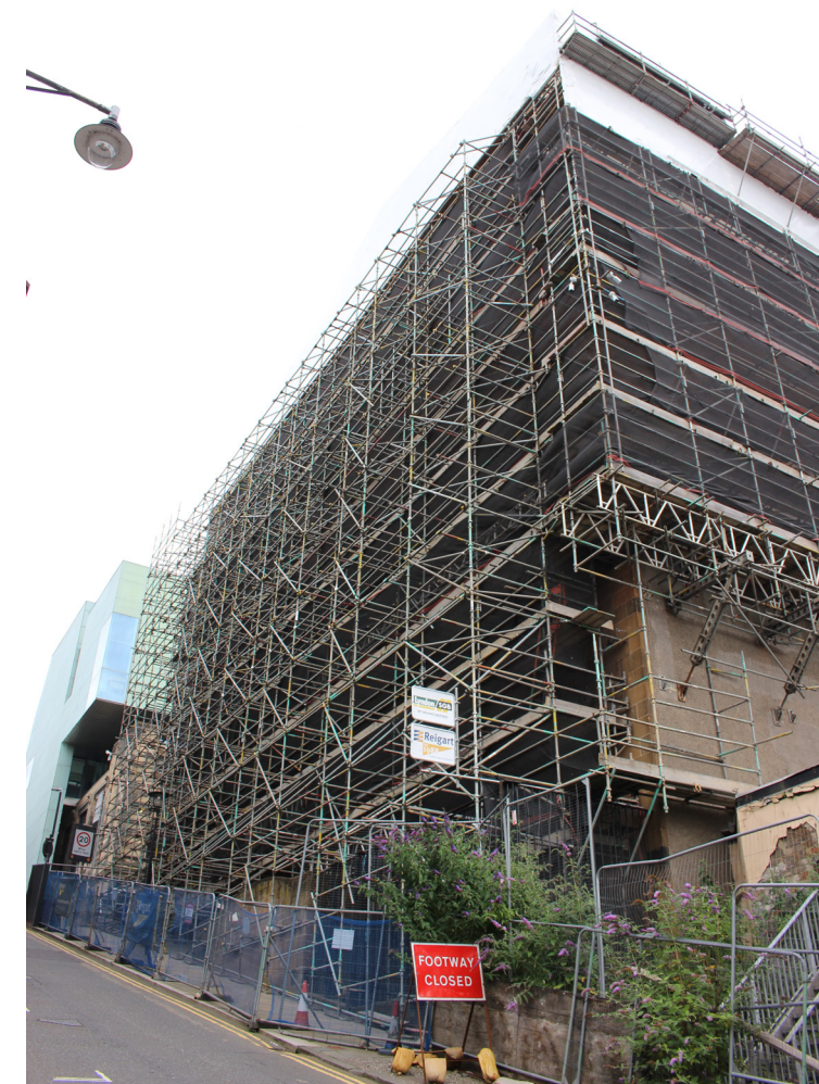
West front of Mackintosh Building
