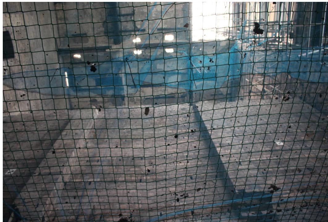
Brick partition walls running to first floor
