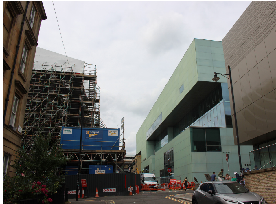
The Reid Building seen from the East
