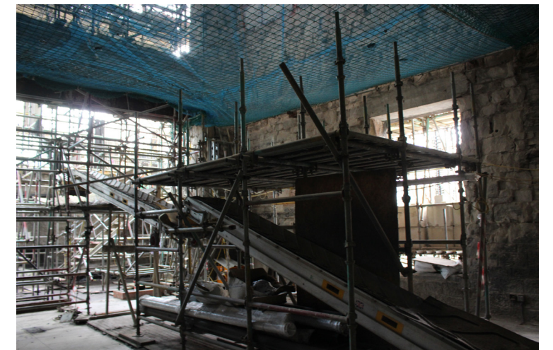
Basement floor of eastern bay showing internal scaffolding
