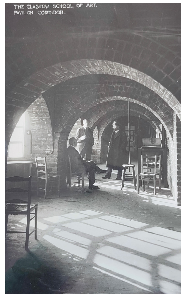
Arched arcade on roof top storey. Glasgow School of Art Archives
