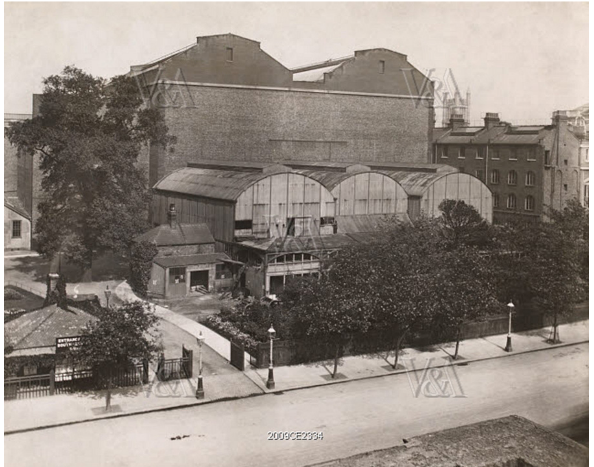
The 'Brompton Boilers', seen in an image of 1897 (E.1038-1989, VAM Collection)009CE2334
