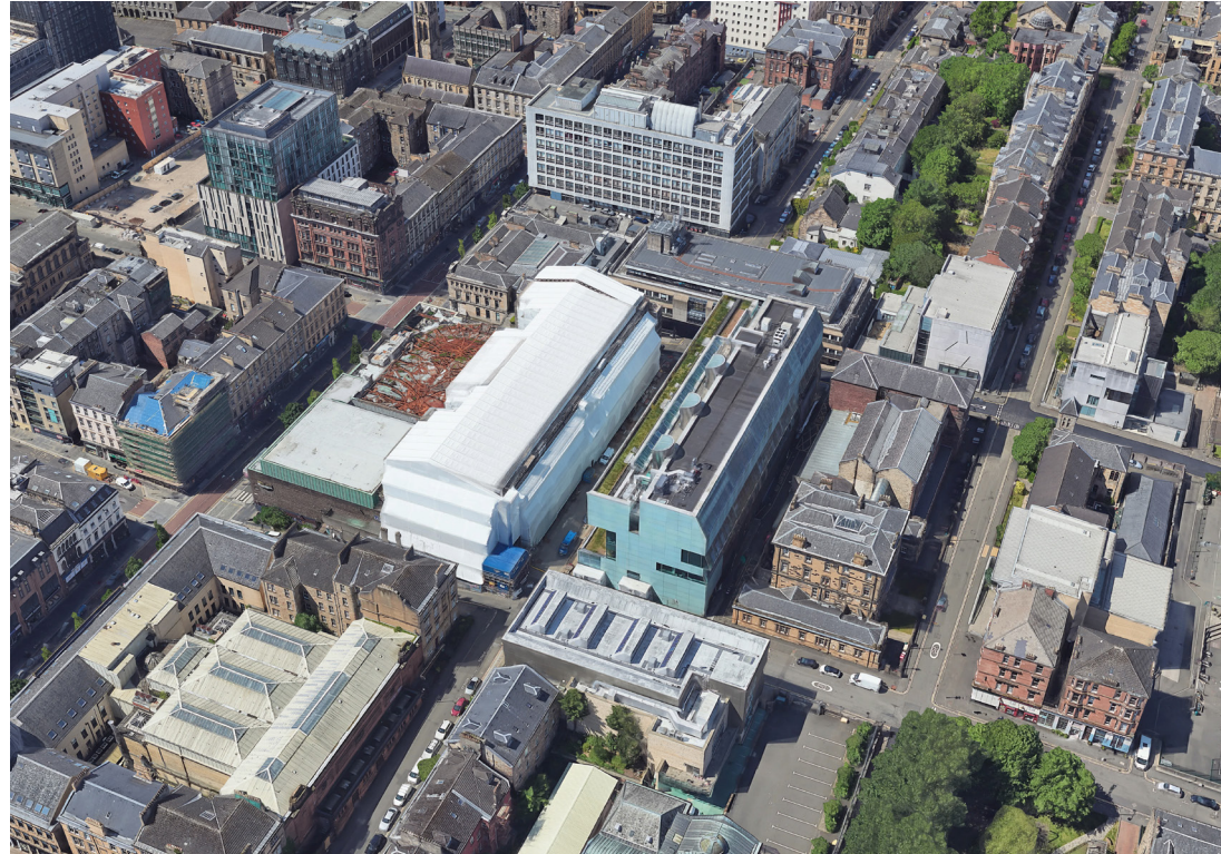
View of the Mackintosh Building looking east and showing the covered scaffolding
