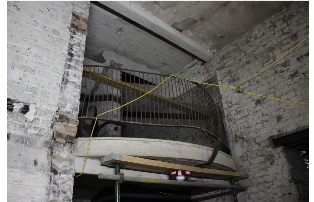
Surviving banister of stair case in central corridor
