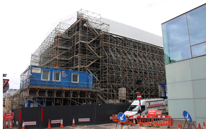
East front of Mackintosh Building, concealed behind scaffolding
