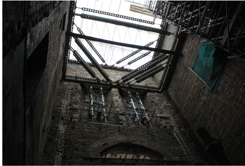
Structural ties within the southern section of the site
