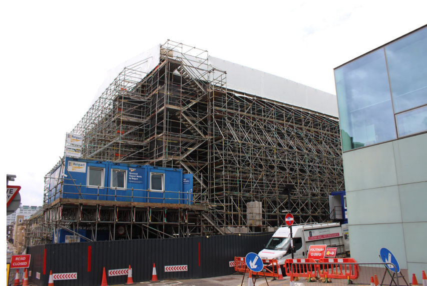
The northwest corner of the building showing the current site office.
