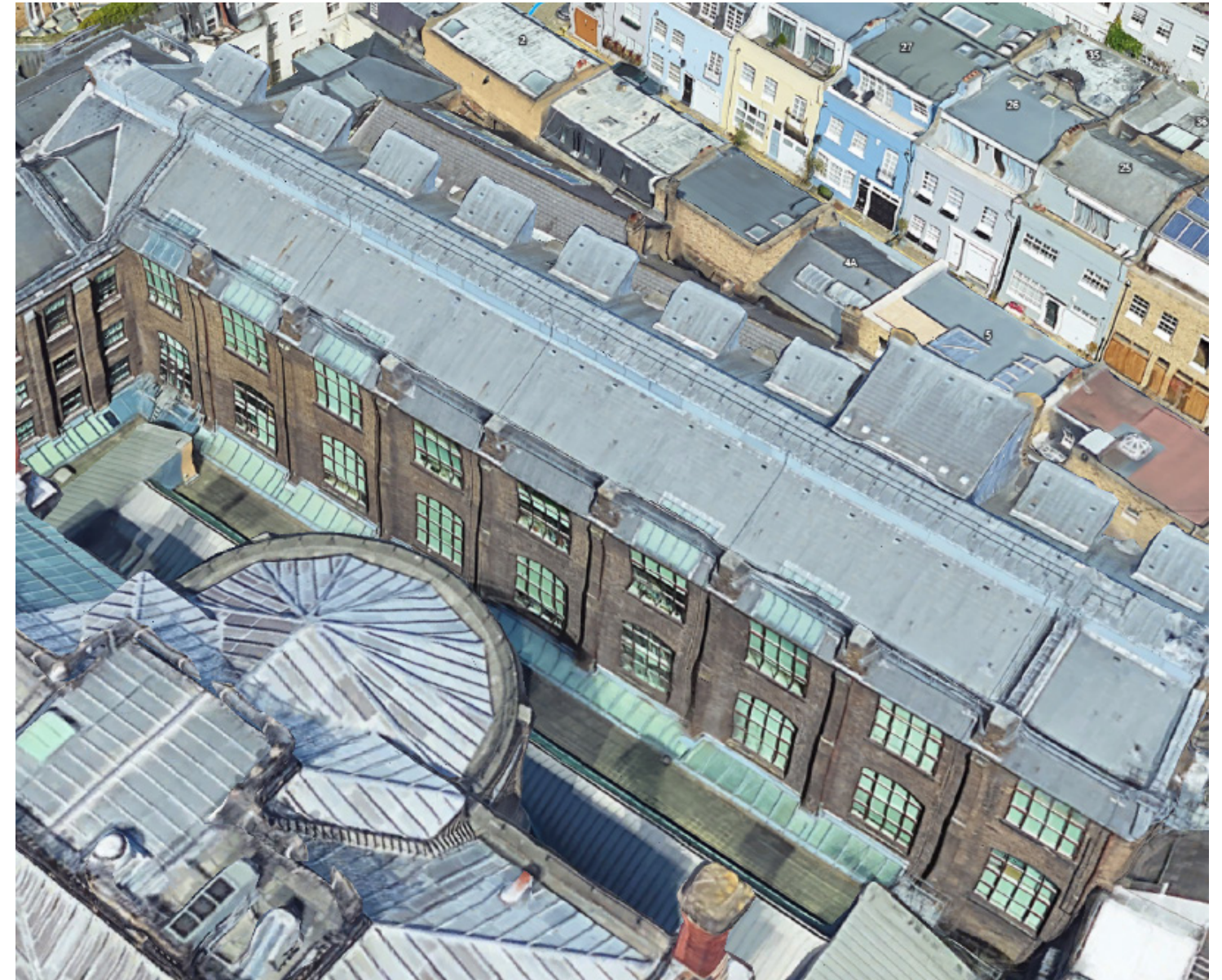
The rear windows at the back of the V&A - a direct precedent for those at the Mackintosh Building.
