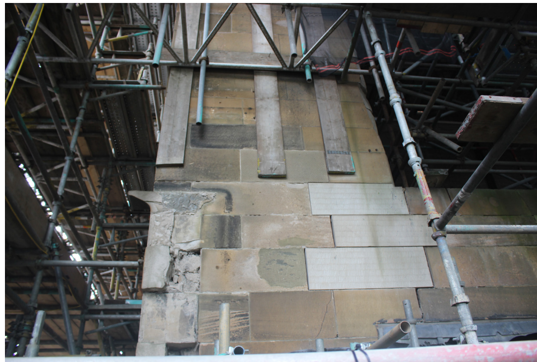
Structural ties along north front
