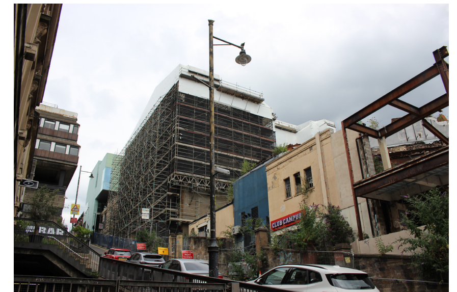
View of the site from the south on Sauchiehall Street with some small visible masonry sections.
