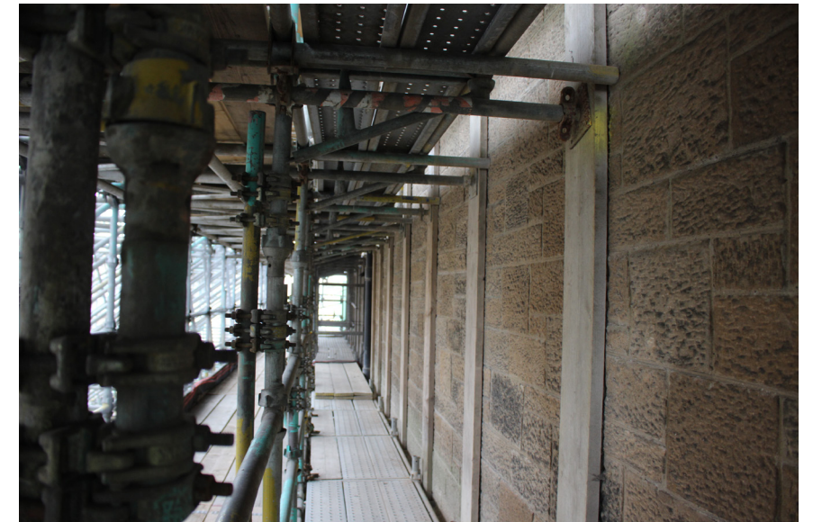
Scaffolding along east front with supporting planks against the wall
