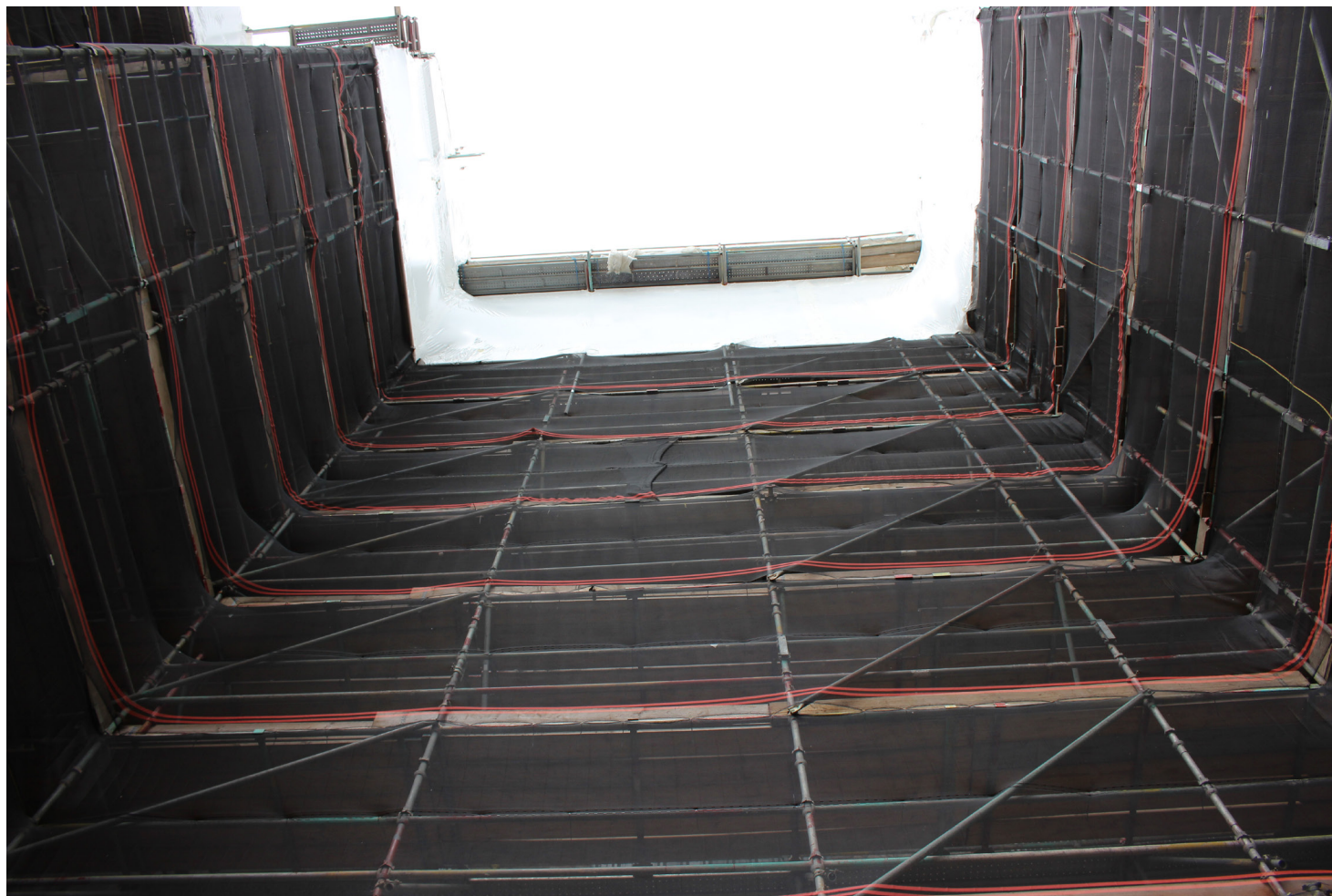
View looking up from internal courtyard on south front
