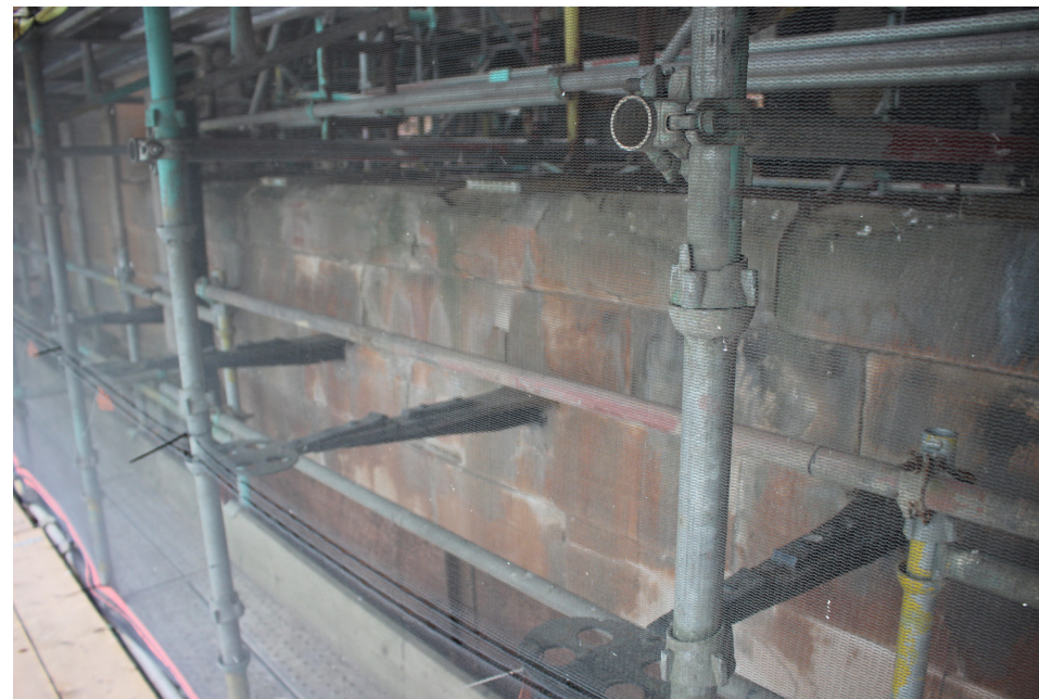
Decorative horizontal hinges survived fire.
