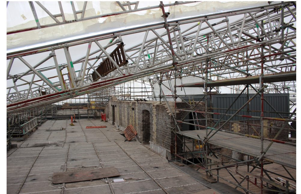
View looking east over ruined roof space
