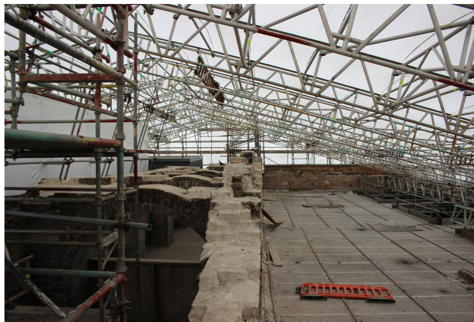
Concrete floor plate in place and arched arcade
