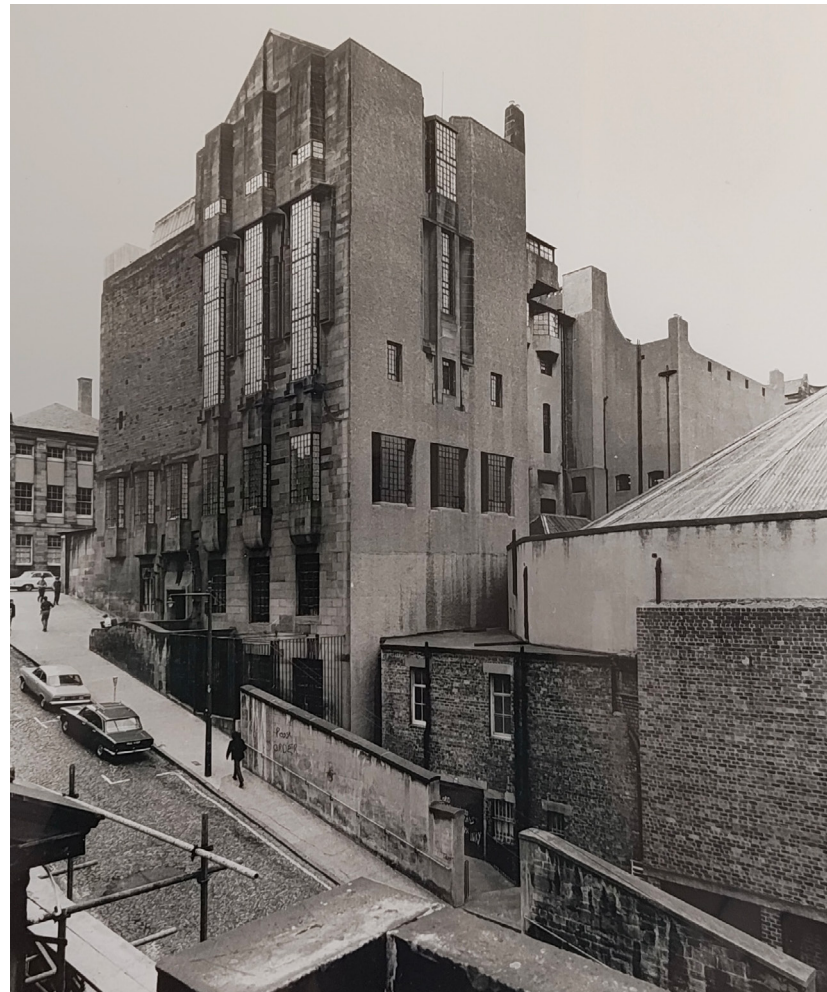
Much celebrated west front and ornate fenestration of southwest corner. GSA A p/7/50
