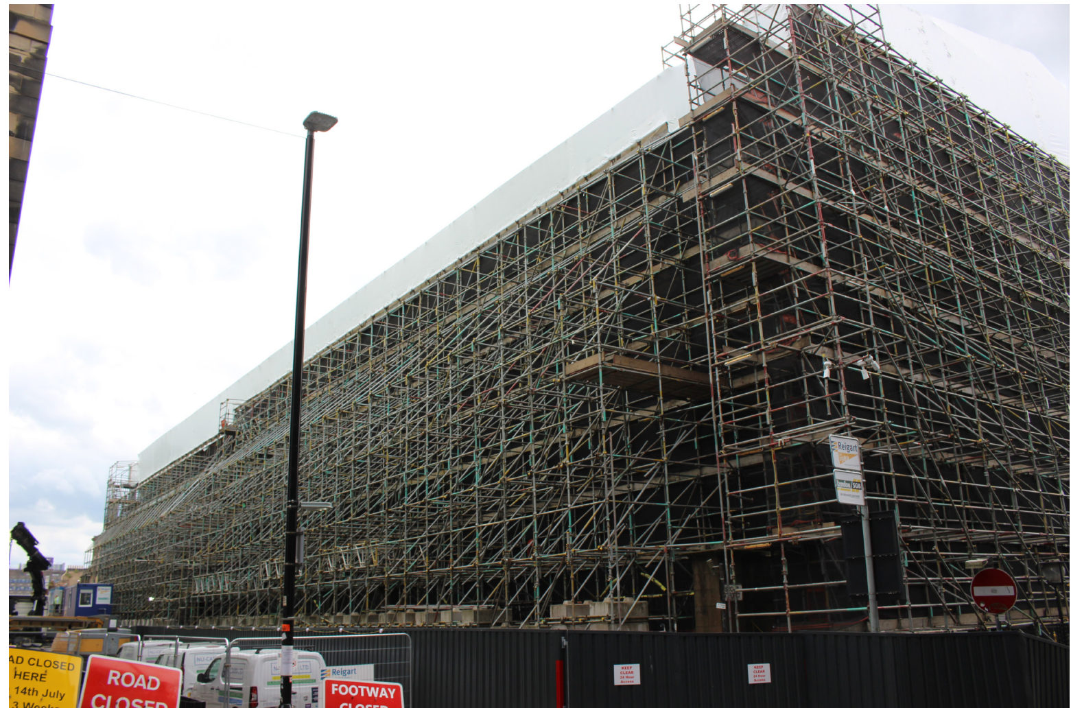
The current extent of the scaffolding, seen looking west along the front façade.
